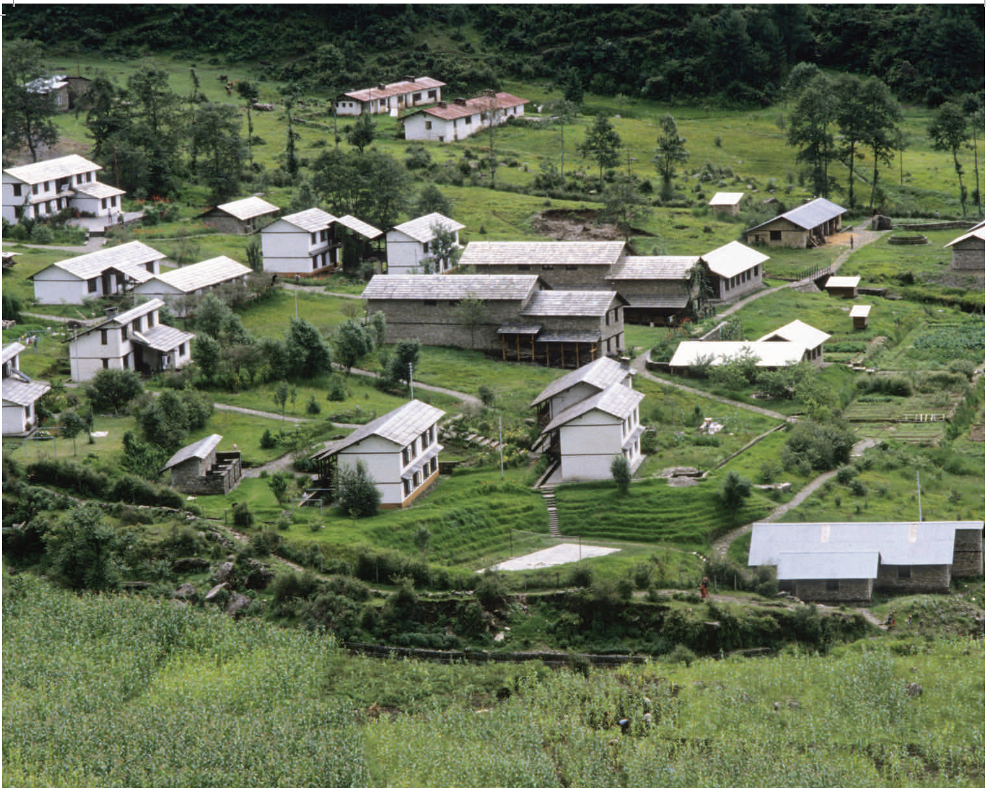
1989. The new compound of the Jiri Technical School (JTS). Built with Swiss assistance, JTS offers two-year courses for junior technical assistants in agriculture, sub-overseers in construction, and auxiliary nurse midwives in health.
